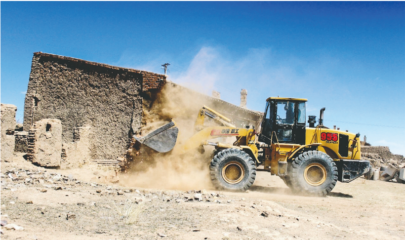
乌兰察布市四子王旗拆旧复垦
