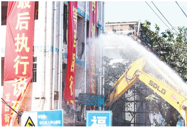
坪山区龙田街道龙兴路拆除现场
